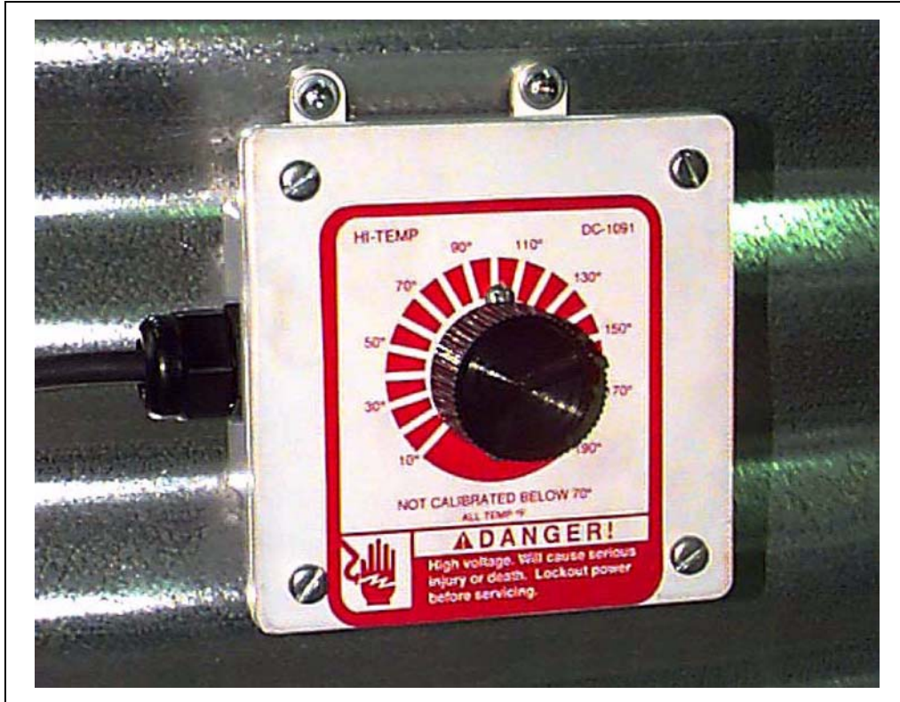
Figure 3E Plenum Thermostat Mounting on Bin Wall
